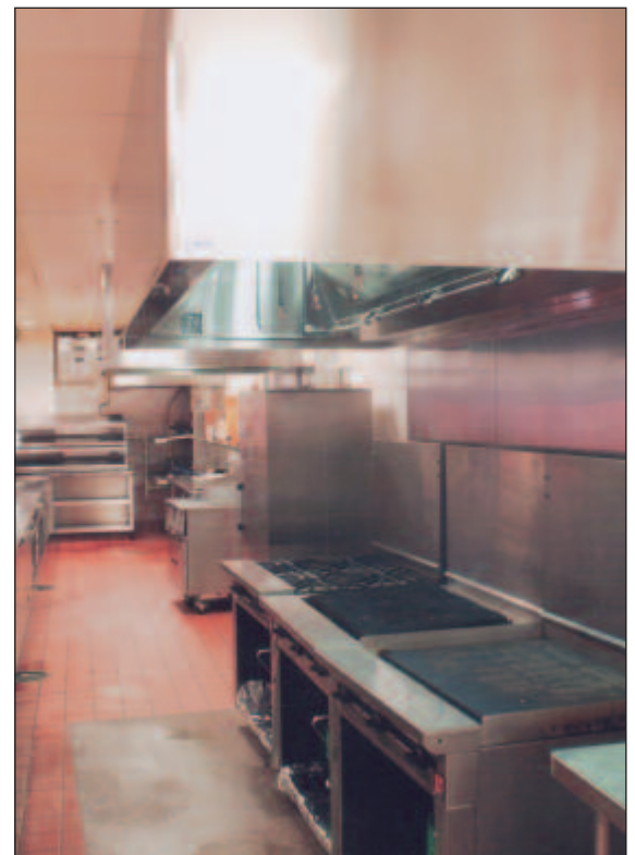
Fifteen new hoods were installed.
