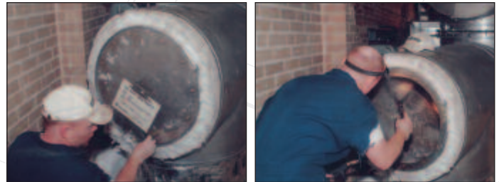
Toolless access panels speed cleaning time. Cleaning process requires no brushing or scraping.
