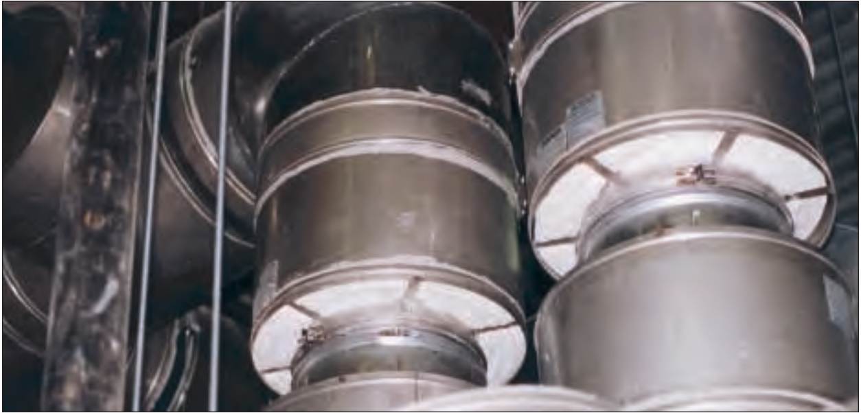
Ceramic insulation and integral steel chase provides maximum temperature control and protection of the insulation.
