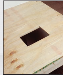
Cut the hole.
