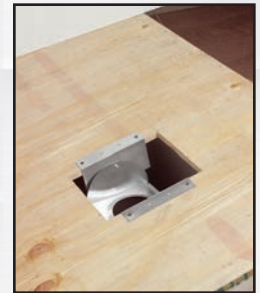
Mount SureGrip support plate.
