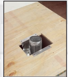
Push pipe through vent support.
