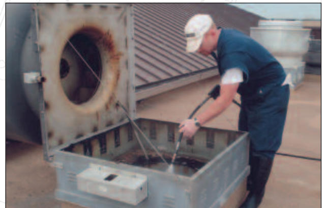
Spraying from roof down, no leaks below.
