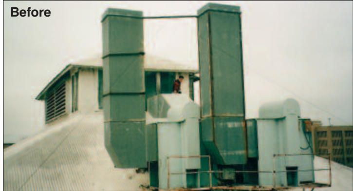
Three large exhaust fans were replaced with multiple smaller fans to serve several smaller cooking and serving stations. This allowed more efficient use, but required multiple duct installations and penetration through already congested areas.
