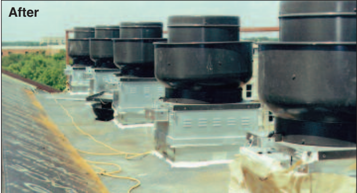
Three large exhaust fans were replaced with multiple smaller fans to serve several smaller cooking and serving stations. This allowed more efficient use, but required multiple duct installations and penetration through already congested areas.
